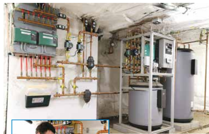
Taco's pre-release System M air-to-water heat pump is installed at the farmhouse, supplying hot water to both the home's large indirect water heater and its main hydronic panel. Left: A technician from Lloyd Plumbing & Heating selects a pumping mode from several available on the Taco 0018e circulator.
