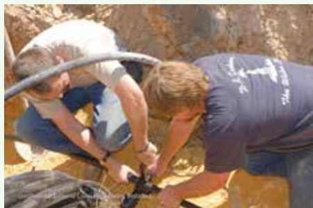
Geothermal ground-loop pipe being installed
