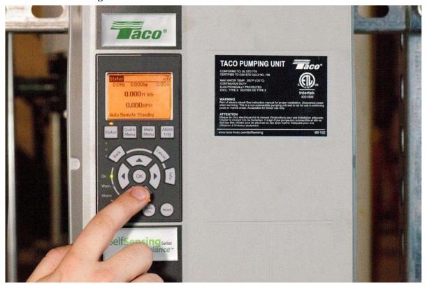
The pumps accurately respond to changes in system demand without the need for pressure sensors. If a classroom zone valve closes, the pumps sense the change and ramp down according to the lower demand. Immediately, the pressure gauge on the supply side starts to drop.
