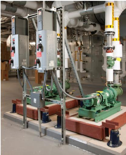
**These drives perform better because of their robust DC link reactor, standard in every SmartDrive® VP. This device offers comparable harmonic performance to AC input reactors without detrimental input voltage reductions, and without the extra heat that would typically be removed via additional fans or other devices.**
