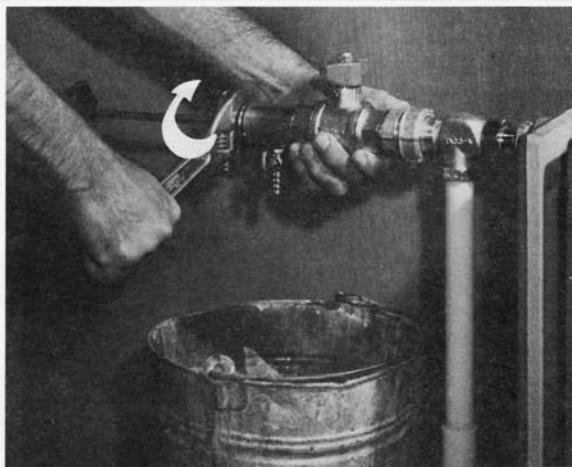
8. Holding the changer so that it does not turn, turn the bonnet out of the chamber.
