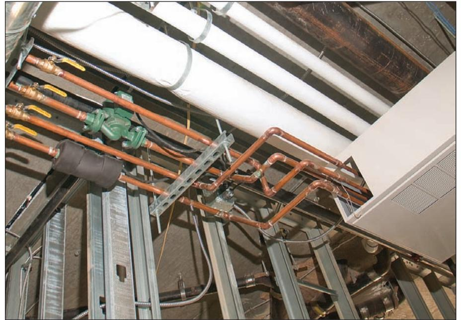
Superior Mechanical Inc. of Randleman, N.C. installed the LoadMatch system using some 350 LoadMatch circulators and Twin Tees throughout the hotel's interior.
