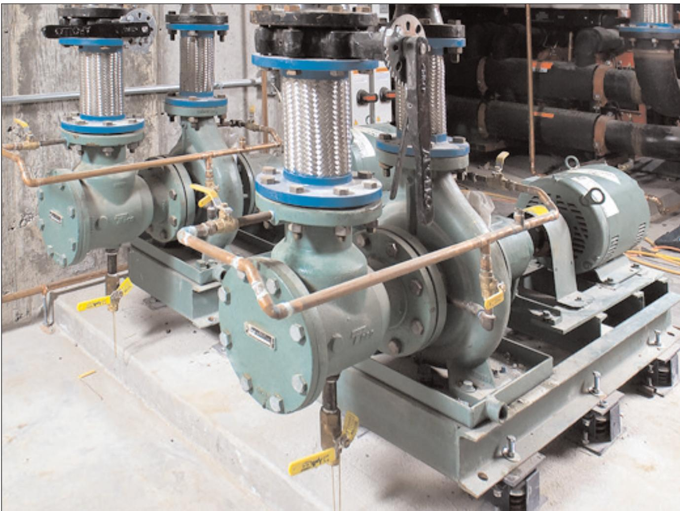
The rooftop mechanical room holds various Taco base-mounted pumps and two gas-fired Raypak modular boilers for redundancy. Using small LoadMatch circulators throughout the system saves on pump horsepower, cutting hp requirements nearly in half.
